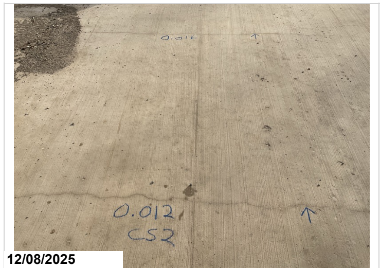
The topside of the deck has 360 SF of minor cracking in various locations, CS2.
