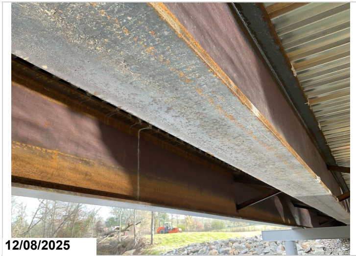
All steel beams speckled rust in various locations.
