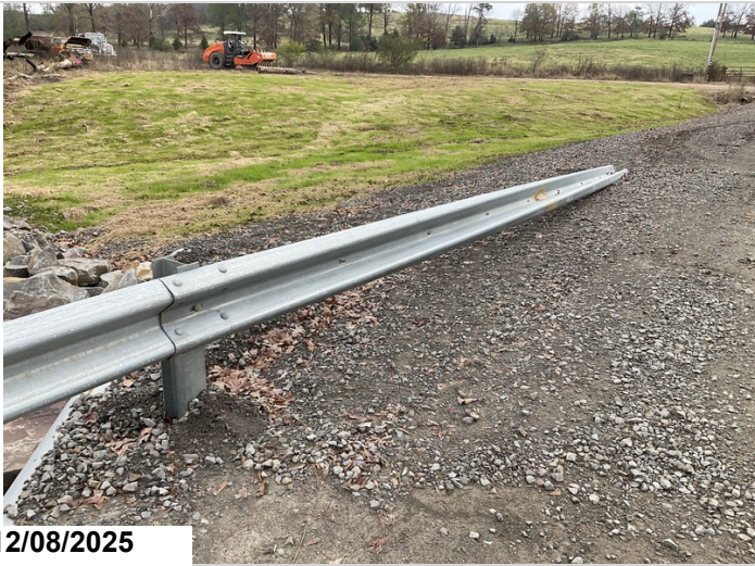
The bridge railing transitions are rated a 9 in this inspection due to no problems being noted.
