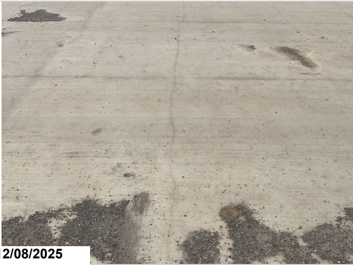
The topside of the deck has 360 SF of minor cracking in various locations, CS2.
