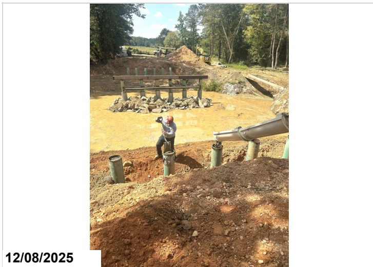
Photo of the concrete being poured into the steel piling.
