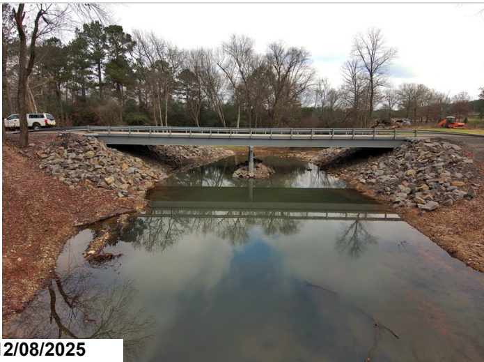
The scour is rated an 8 in this inspection due to riprap being placed around both ends of the streambank.
