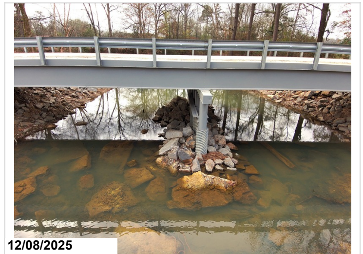
Channel protection around bent 2.
