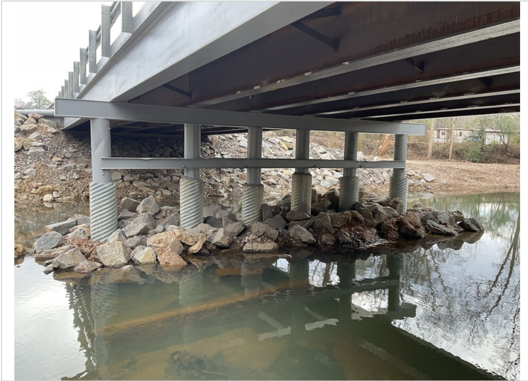
Bent 2 steel cap NSTM member
