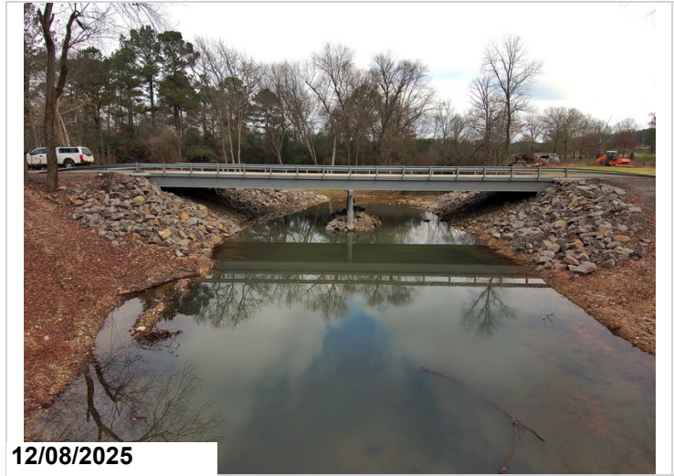
The channel protection is rated a 9 in this inspection due to riprap being placed around both sides of the streambank.
