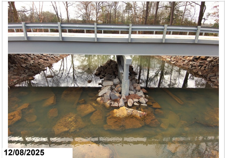
Channel protection around bent 2.
