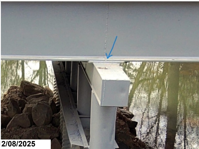
Photo shows cover plate and bearing area welded to bottom flange at center bent.
